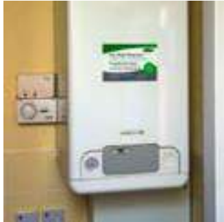
Wall Mounted Gas Boiler
